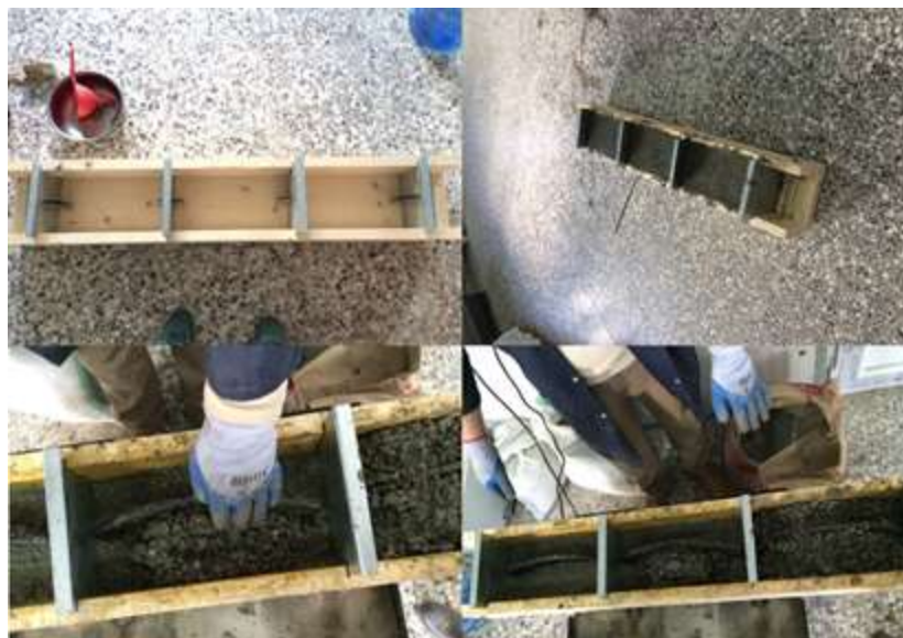
Figure (2) Thermal resisting concrete blocks casting.
