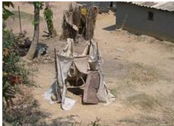
Figure 3: Pit latrine without slab in Lusaka, Zambia
