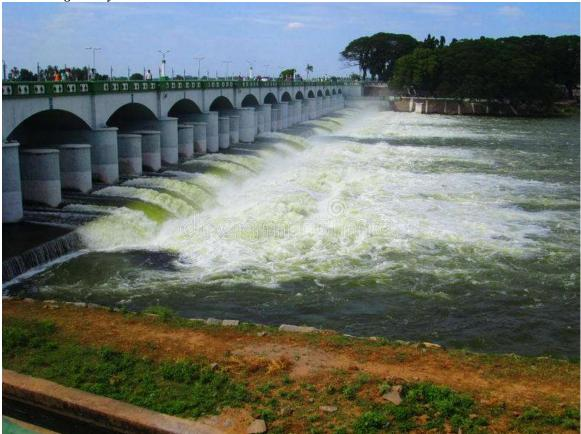
A dam made in a stream for maintaining and regulating irrigation. Anicuts are used to maintain required water level in the upstream by releasing only the excess water to downstream. In the lifting gate, water is allowed to flow from the bottom and this causes high erosion in the canal.
