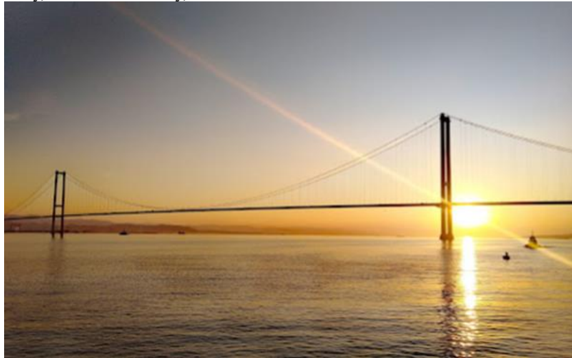
Photo 4: Osman Gazi Bridge
