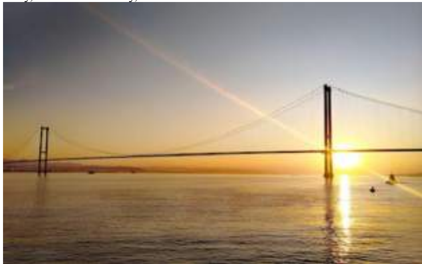
Photo 4: Osman Gazi Bridge
