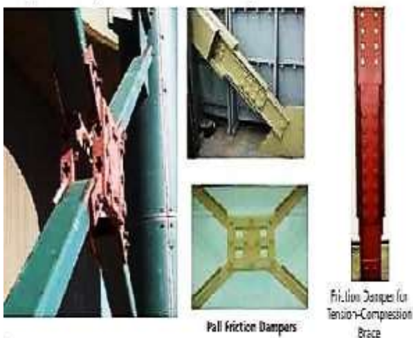
Figure 3: Friction Damper
