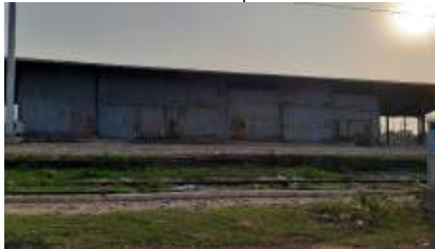
Figure 4: Railway storage from 19 th century
