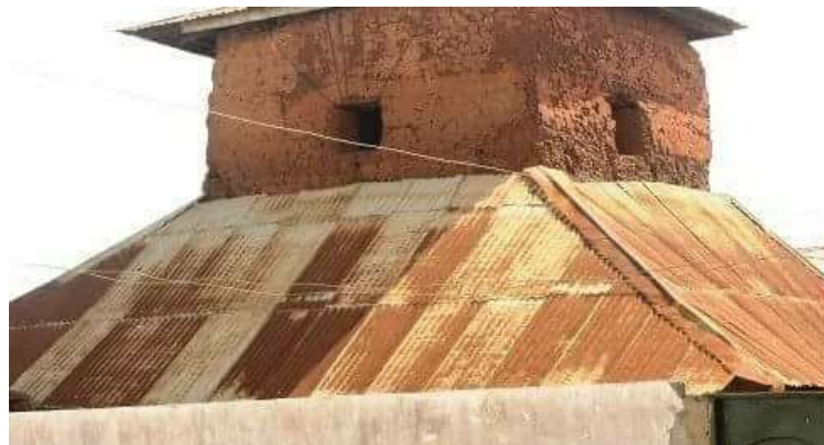
Figure 9: Odogo tower, located in Idah, Kogi State
