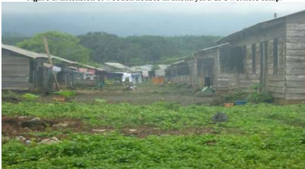
Figure 1: Extension of wooden houses in Ekona yard CDC workers camp.
