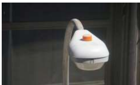
Fig. 1. Illumination Sensor on a Gas-Discharge Luminaire
