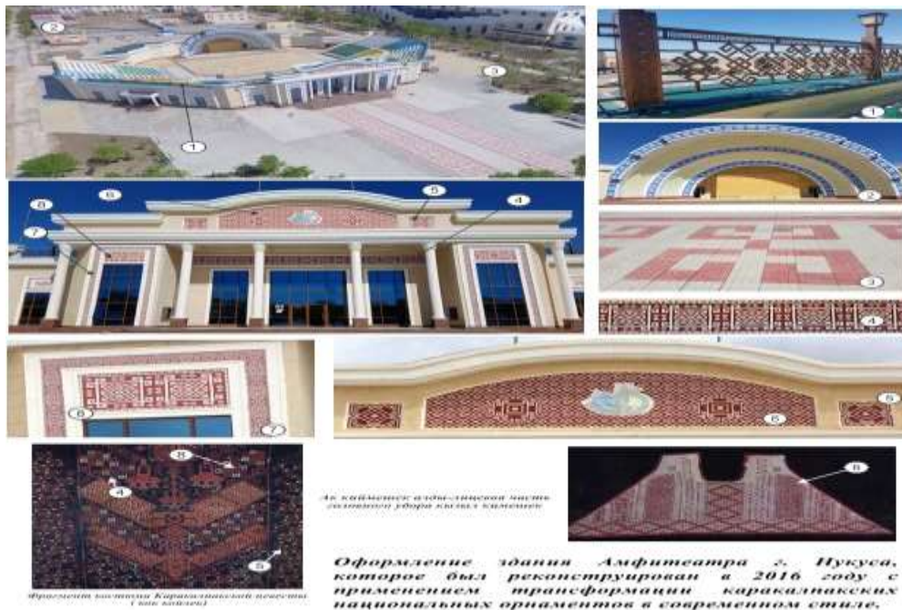
Fig. 6. Buildings of the Amphitheater in Nukus after reconstruction
