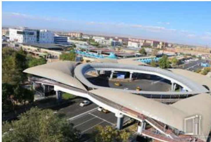
Figure 5. Construction of an underground mega-bridge for pedestrians in Navoi
