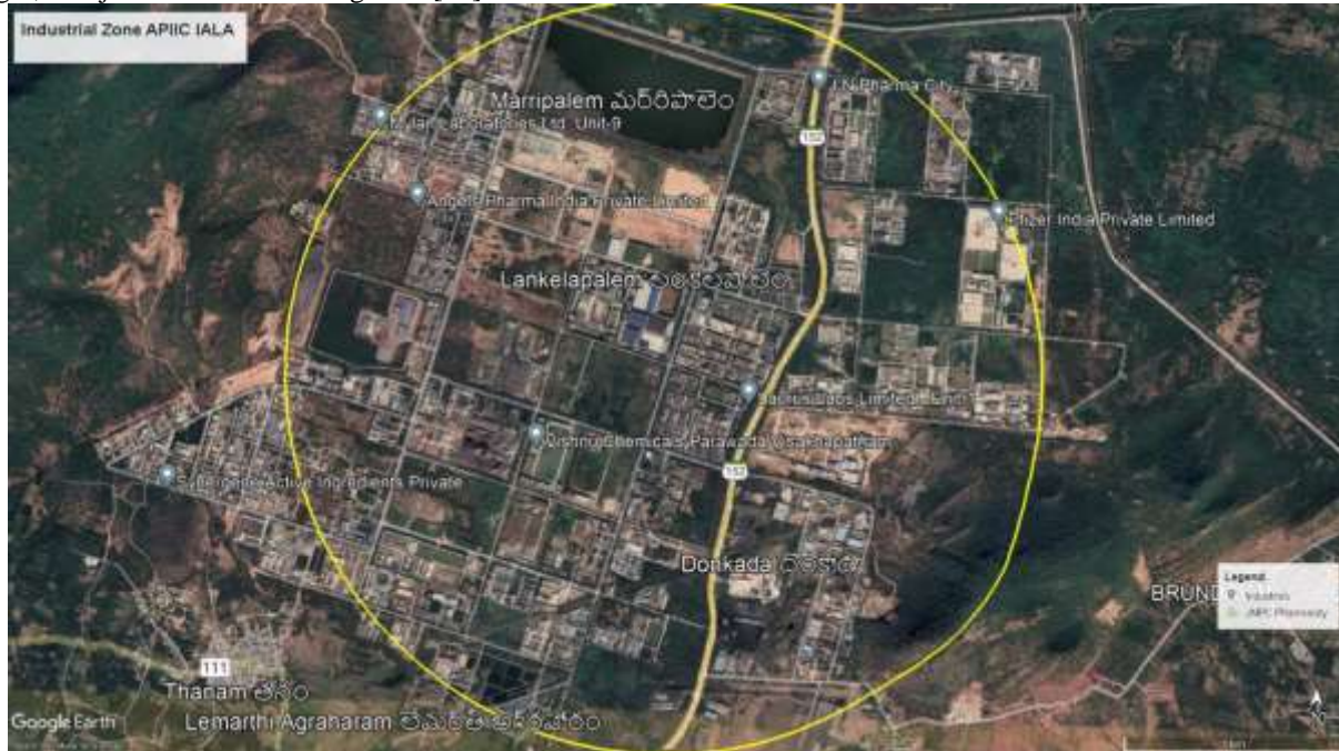
Fig. 6 Google Earth image of the Industrial Zone, APIIC, Parwada, Vizag (A.P.)
