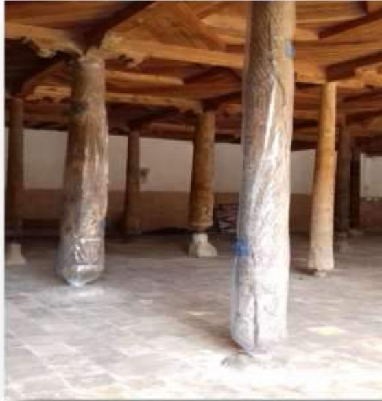
Figure 1: Method of collecting Hylotrupes bajulus, a black house beetle of the genus Hylotrupes, from museum columns.
