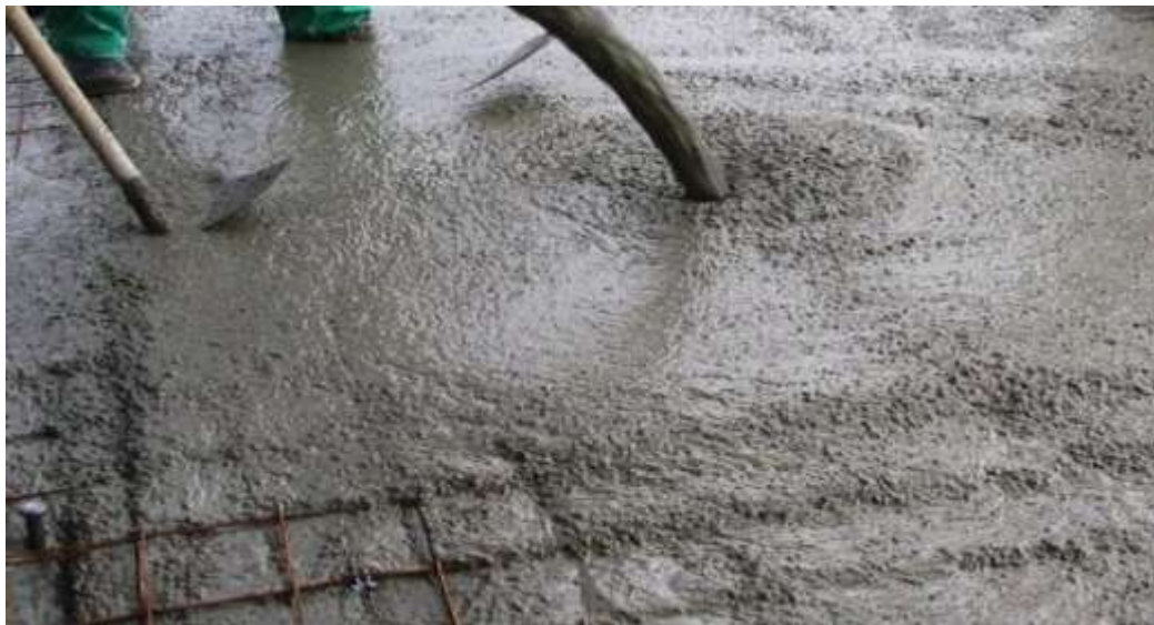
Fig 1: Flooring Finish done by self compacting concrete
