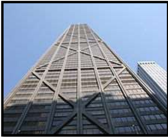
Fig-3: Cross- bracing
