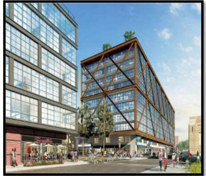
Fig-1: Exoskeleton Structure with X-bracing in London
